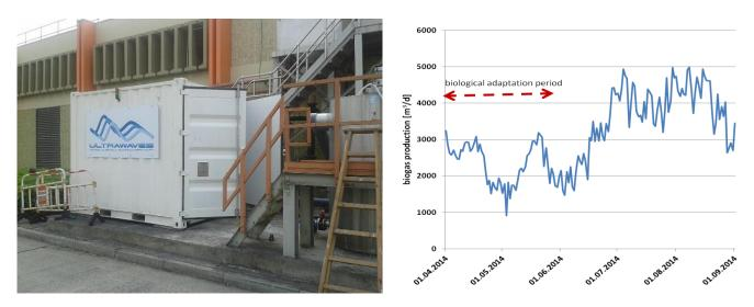
Figure 3: Demo Installation at Shek Wu Hui STW. A 5 kW ULTRAWAVES ultrasound reactor unit as plug&play system in a 10<sup>-</sup>-conatiner is operating since April 2014. After the typical adaptation period we can observe an increase in biogas production.
