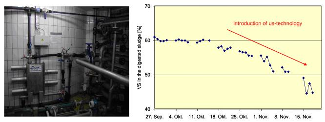
Figure 1: Installation at Meldorf WWTP and results. The volatile solids (VS) in the digested sludge were significantly reduced in conjunction with the introduction of ultrasound technology at Meldorf WWTP. Analyses reveal that the VS content of the digested sludge was reduced from 60% to 45% over the course of the test period.
