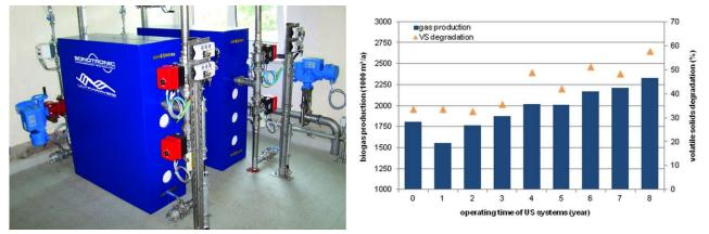
Figure 2: Installation at Bamberg WWTP and results. By using the ULTRAWAVES ultrasound systems the degradation of the organic sewage sludge components was increased from 34% at the beginning to more than 50%. At the same time the biogas production was increased by more than 30%.
